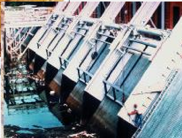
Figure 269. Rack and pinion bar screens.
