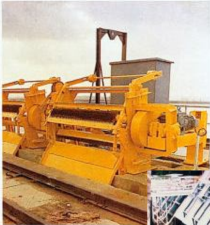
Figure 268. Fine bar screens (GFD)
