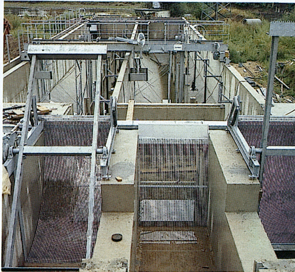
Figure 264. Curved bar screen (DC type).
